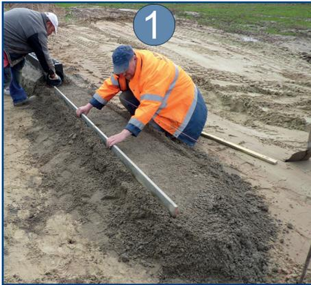
The concrete bed is laid in accordance with the necessary load class to install the HYDROblock.
