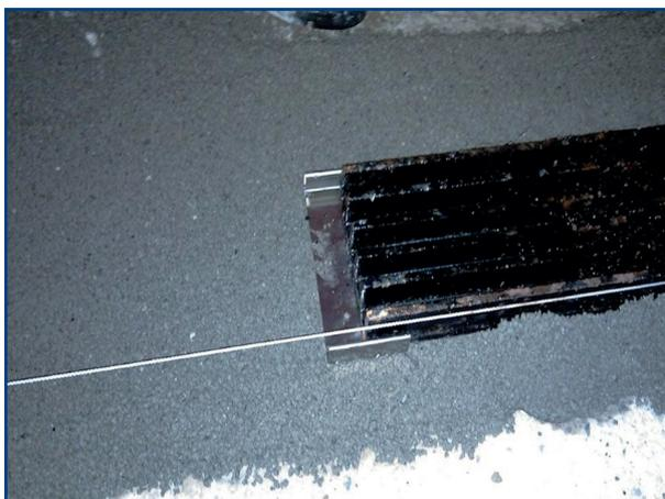
The channel must be seated at least 3mm lower than the adjoining surface.
