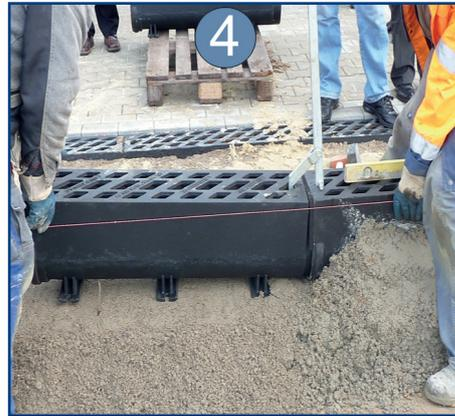
The HYDROblock laying tool is then used to pull the elements together.
