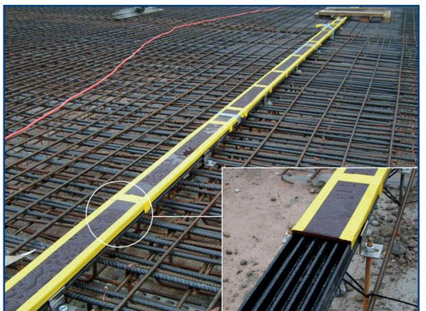
Before laying down the concrete layer the flat channel must be covered and taped to prevent the ingress of concrete.
