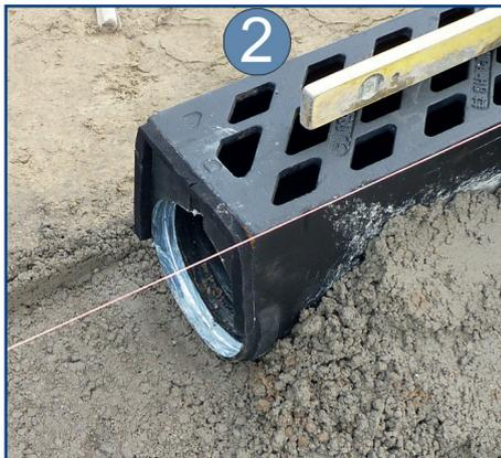
Before the elements can be joined, apply a lubricant to the spigot.
