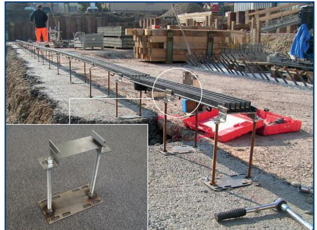
The installation supports must be placed at the joints of the HYDROline. In this case we also recommend placing end sections at the beginning and end of the channel.
