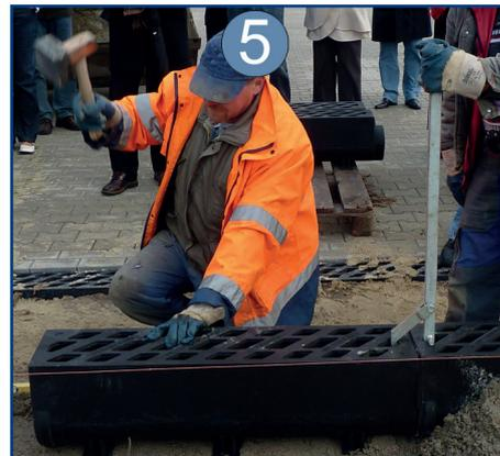
After connection the element is set at the correct height.
